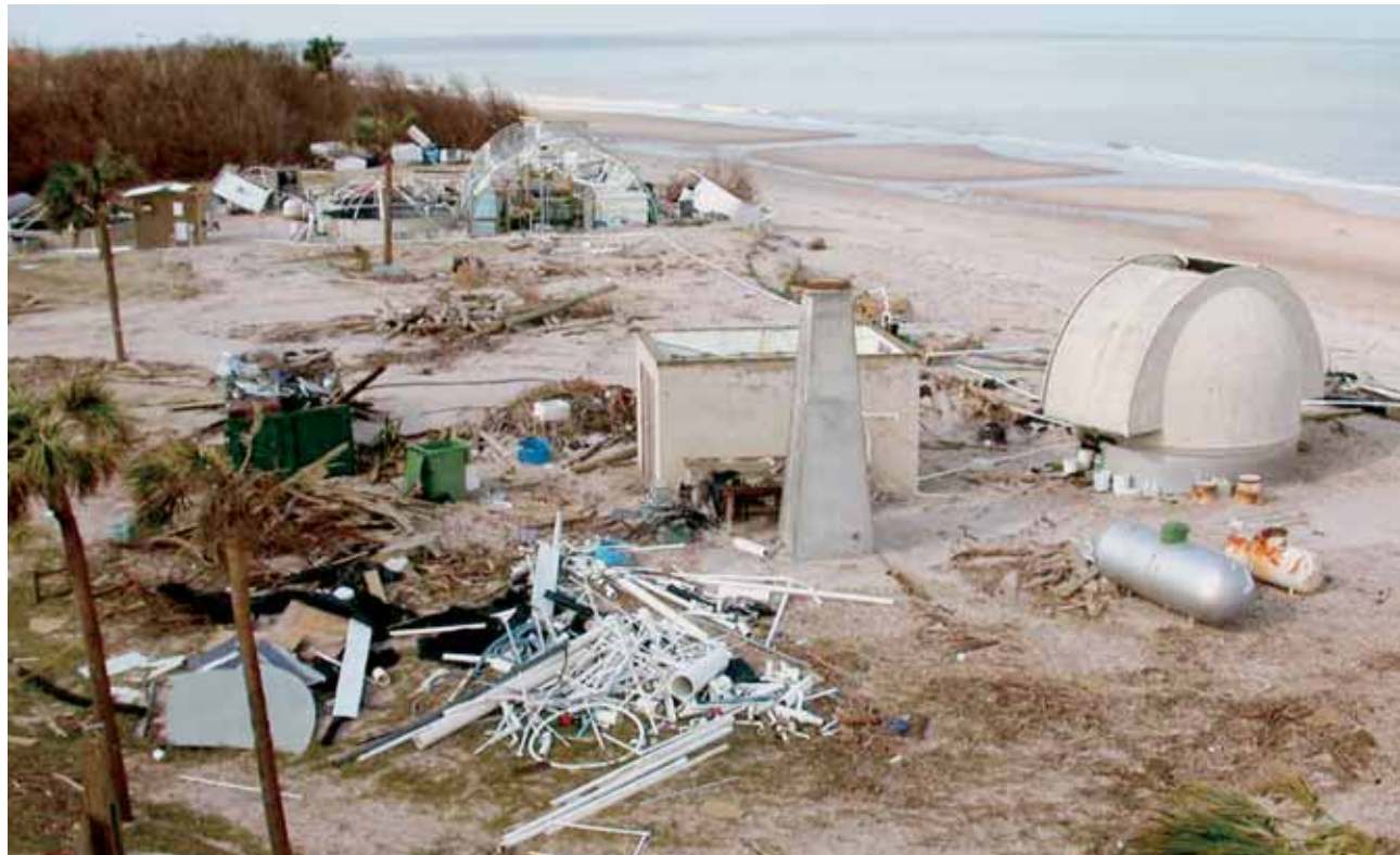
The Vero Beach Marine Lab facility suffered extensive damage from wind and water.
