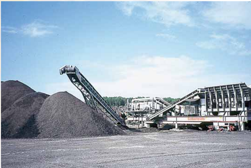
The RAP crusher goes to work during post milling processing to resize the RAP for use in recycling.
