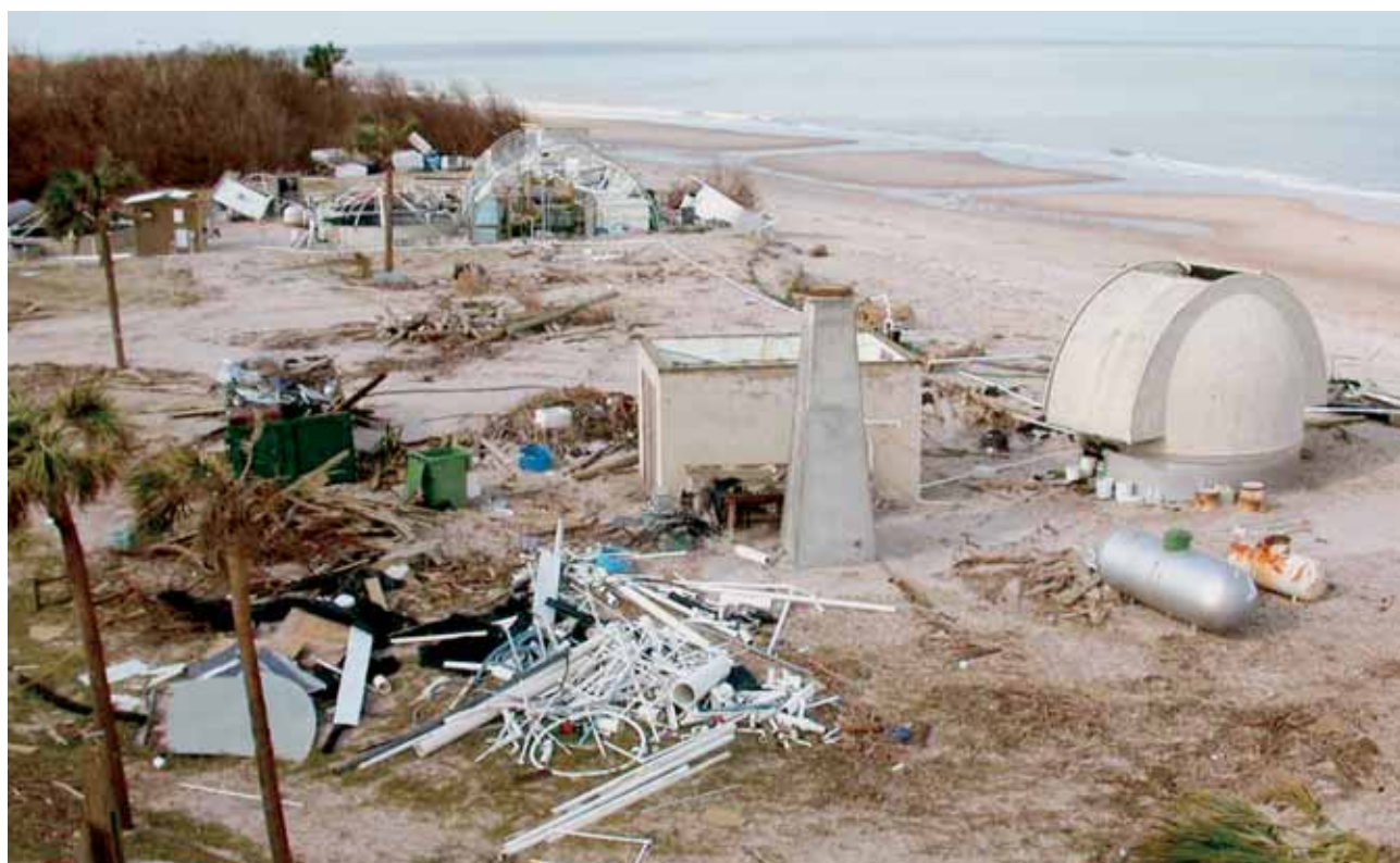
The Vero Beach Marine Lab facility suffered extensive damage from wind and water.
