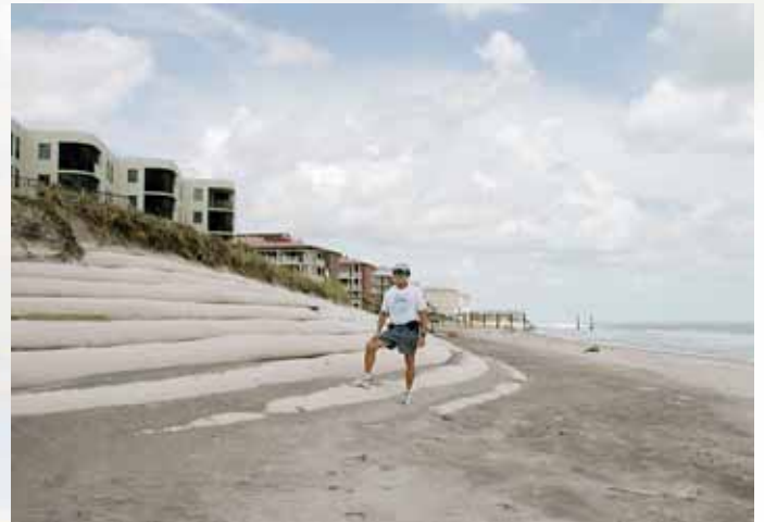
Dr. Lee Harris visits Vero Beach in September 2004, inspecting an experimental sand-filled container revetment system that successfully provided coastal erosion protection during the hurricanes. He was the design engineer and oversaw the project construction during the summer of 1989, for the system noted by the Florida Department of Environmental Regulation (FDEP) for its successful performance.
